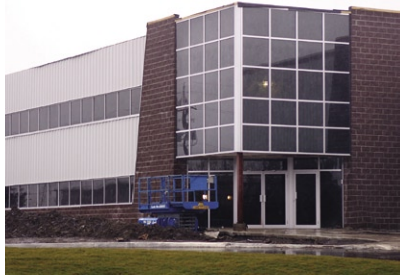
The Robinson Group's new corporate head office
